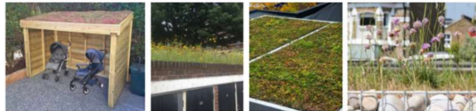
3 New buggy stores and bin stores with green roofs for water management and wildlife benefit.
